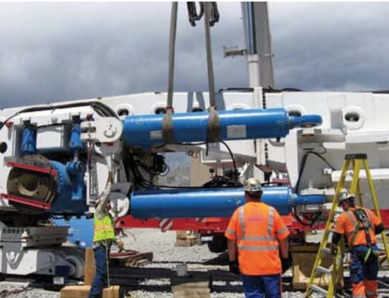
Crews load the TBM onto specialized transport dollies for final assembly in a launch chamber
