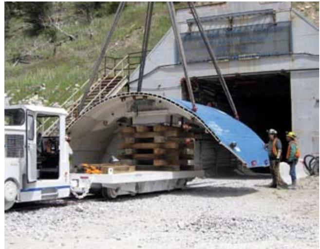
Crews ready the roof shield of the TBM for transport through the small portal area, just 4.1 m high and 4.4 m wide
