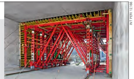
VARIOKIT, the engineering construction kit with rentable, standardised components, is the solution for numerous requirements in tunnel construction.
