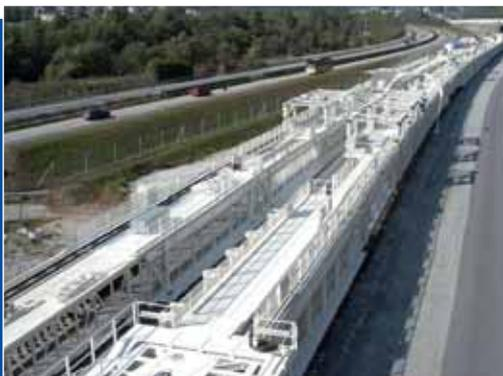
Innerlining system „The Worm“ , Gotthard base tunnel, Switzerland
