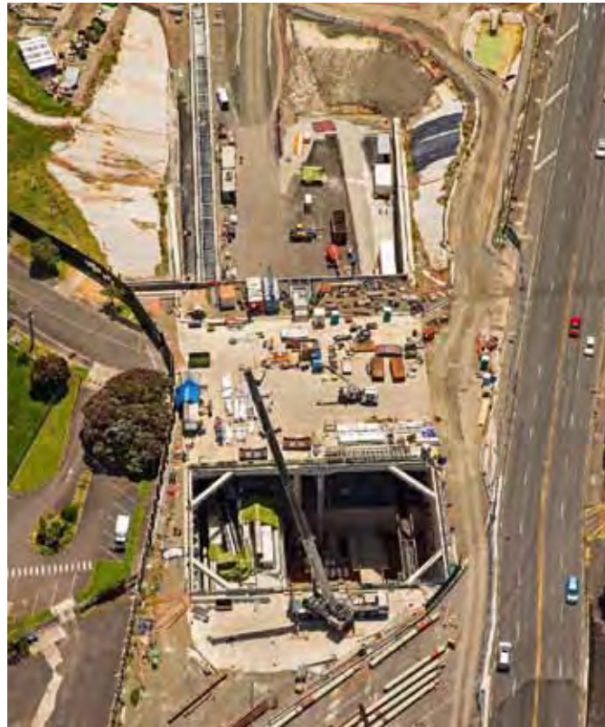
6 After breakthrough on 29 September 2014, the machine had to be turned around and pushed sidewise in the northern portal trench to start the excavation of the second bore in the opposite direction
