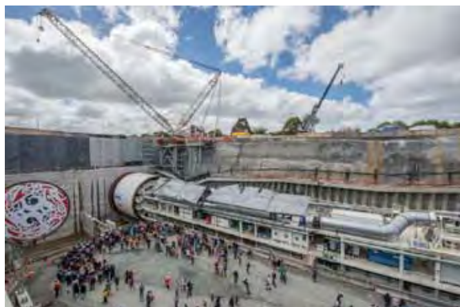
5 The EPB shield has an overall length of 87 m including backup gantries. The machine was ready to bore the first tunnel section on 31 October 2013
