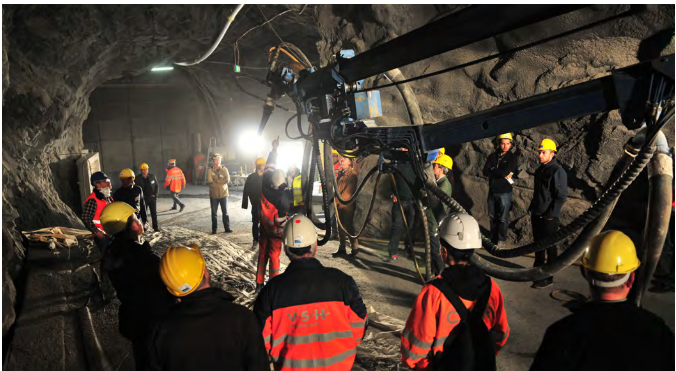
Quelle/credit: Versuchsstollen Hagerbach AG
