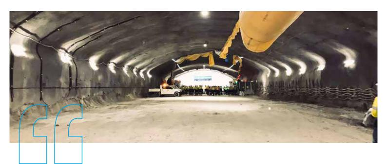
In what is described as one of the most complex underground junctions ever built, WestConnex is a 33-kilometer (21 mi) predominantly underground motorway tunnel network in Sydney. Its walls are lined with two permanent sprayed layers: one is a fiber reinforced primary support lining, the other is a fiber reinforced concrete smoothing layer. Both are reinforced with Dramix® 4D steel fiber for optimal load-bearing capacity.
