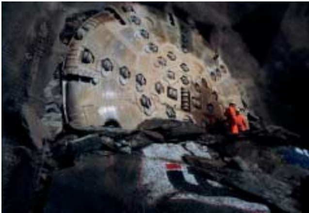
4 Durchschlag der TBM in Sigirino 4 TBM breakthrough at Sigirino
