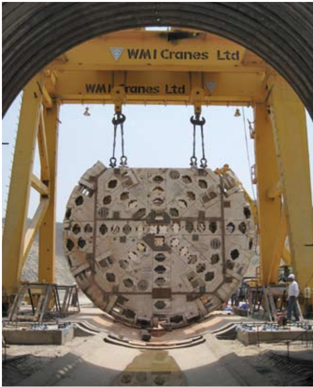
The Double Shield TBM for India's Veligonda Water Tunnel was assembled at the jobsite in 2009, using Onsite First Time Assembly (OFTA)
