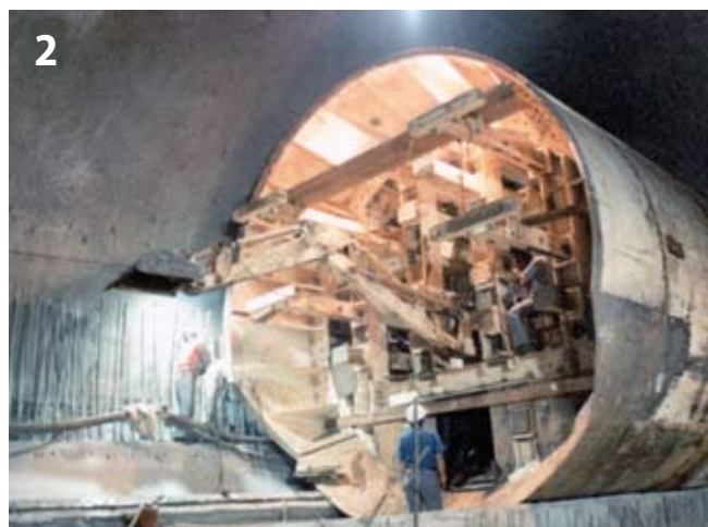
Single-track open face TBM used for the São Paulo Metro Line 1 in the 1970s
