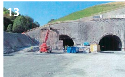
Violay-Tunnel Violay Tunnel
