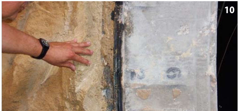
Verpresster Ringspalt Grouted annular gap
