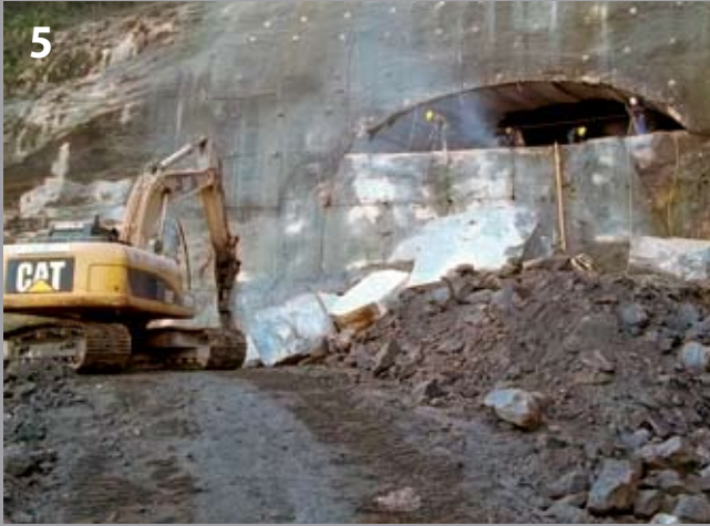
Opening of the tunnel mouth in Barra da Tijuca
