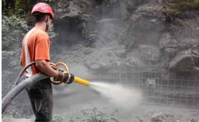
The Aliva Converto is used for hand-operated spraying of concrete and mortar, applies with thin and dense stream process. The new water ring system can be easily assembled and allows a simple transition from dry to wet spraying applications when the thin stream process is used. The modularly based concept allows the operator to assemble four different types of spraying-tools: the Converto spraying device,
